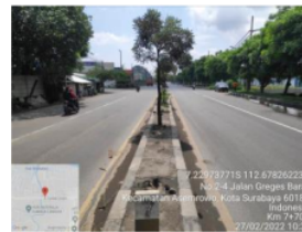
Figure 3. Condition of Jl. Gresik KM 7+700
