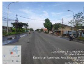
Figure 2. Condition of Jl. Gresik Km 4+900
