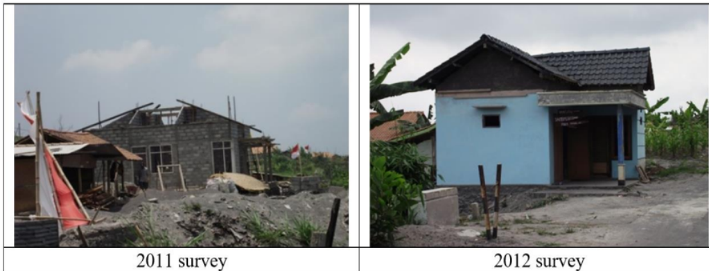
Figure 1. Independent House Construction
